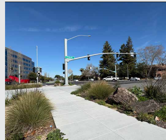
Curb Extension at Mathilda and Maude avenues
